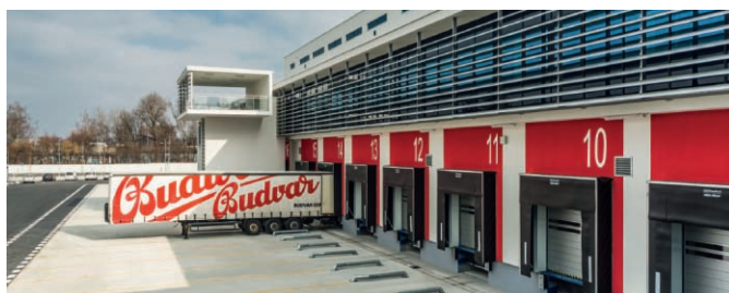
The floorless operation of the high-speed doors is vital to Budweiser Budvar
