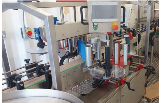
The complete system has been installed in a specially adapted container
