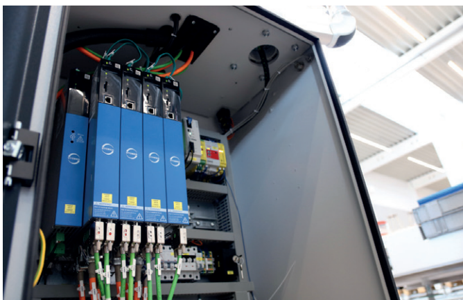
The SI6 drive controllers from Stober Drives save space in the control cabinet
