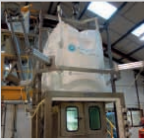
Containment of material is key
