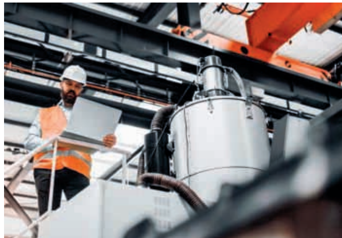
This standalone system can be extended to cover additional machinery
